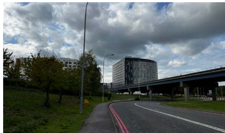
Figure 86. Perimeter Road North view towards NT Hotels
